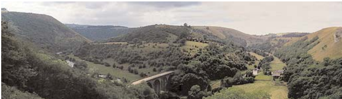
Viewed from Monsal Head, the Monsal Trail passes over Headstone Viaduct, and then on towards Millers Dale
